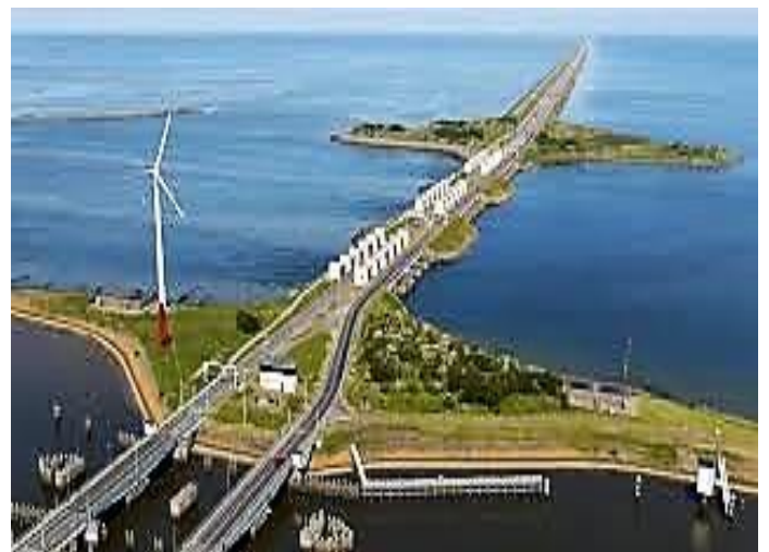
The Western On-ramp to the Afsluitdijk
