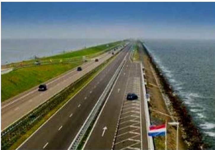
The 32Km man-made dyke with 4 lanes
