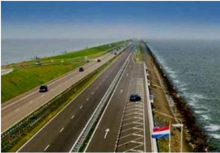
The 32Km man-made dyke with 4 lanes
