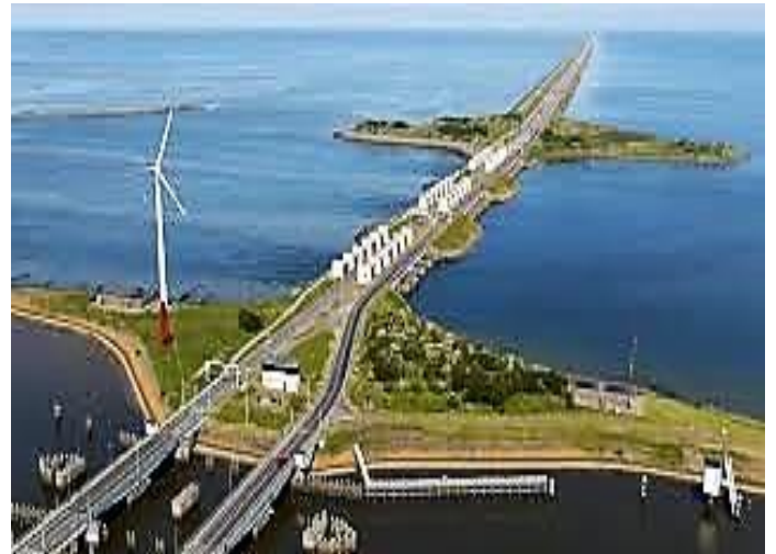
The Western On-ramp to the Afsluitdijk
